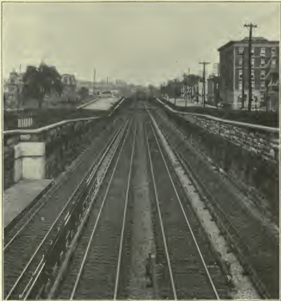
FIG. 506. THIRD RAIL CONTACT SYSTEMS. Main Track Construction, 600 - Volt Under Running Third Rail Installation, New York Central & Hudson River Railroad, New York City.
